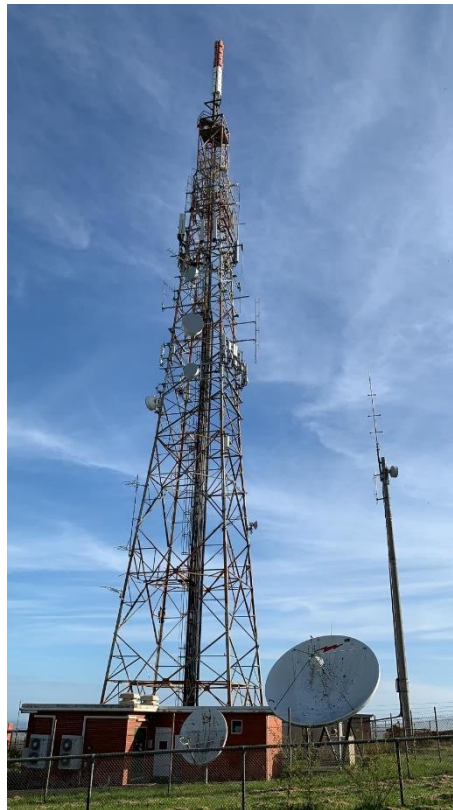
Figure 3-1 Tower Hill – Transmission Tower
