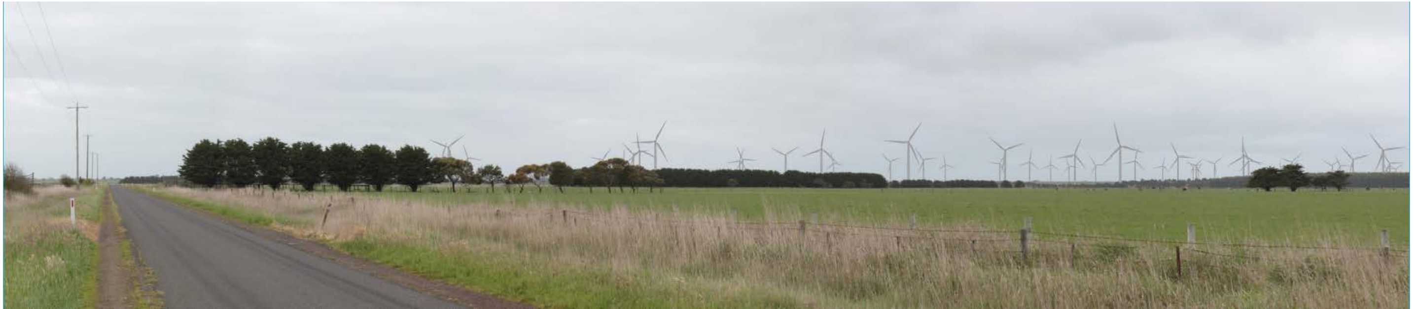
Figure 6-5 Viewpoint RC02 - Photomontages showing the Approved Layout (above) and the Amended Layout (below)
