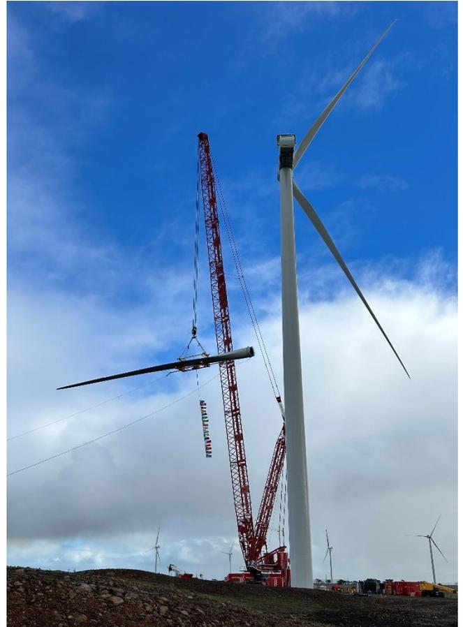
The last blade is lifted in place. A flag was attached to the cable for each nationality involved in the construction.
